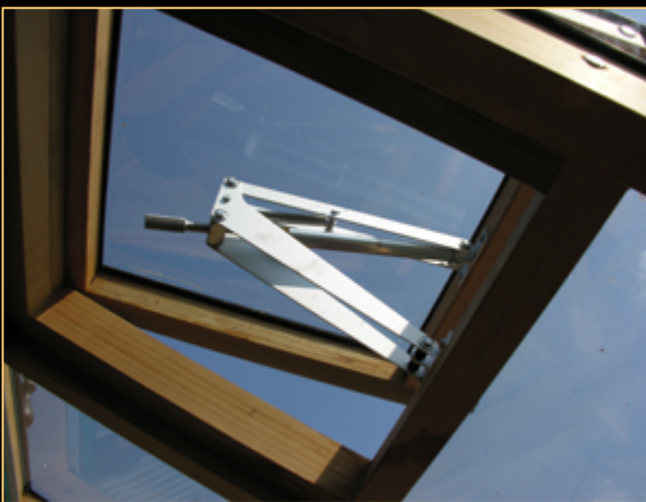
Above picture shows a triple spring autovent
