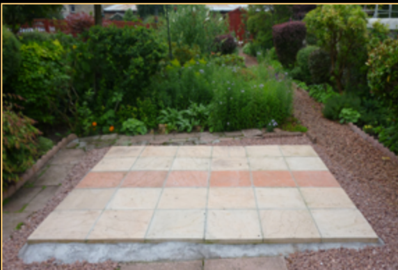
Example slabbed base for a cedar greenhouse
