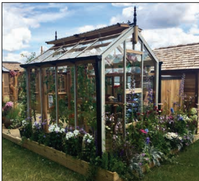
Rear gable and side elevation fitted with aluminium cladding
